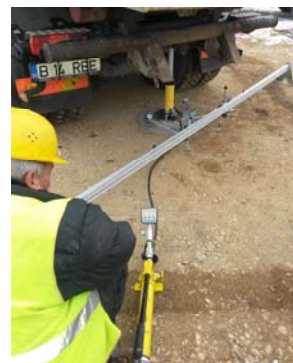
Fig. 2. Plate bearing test
