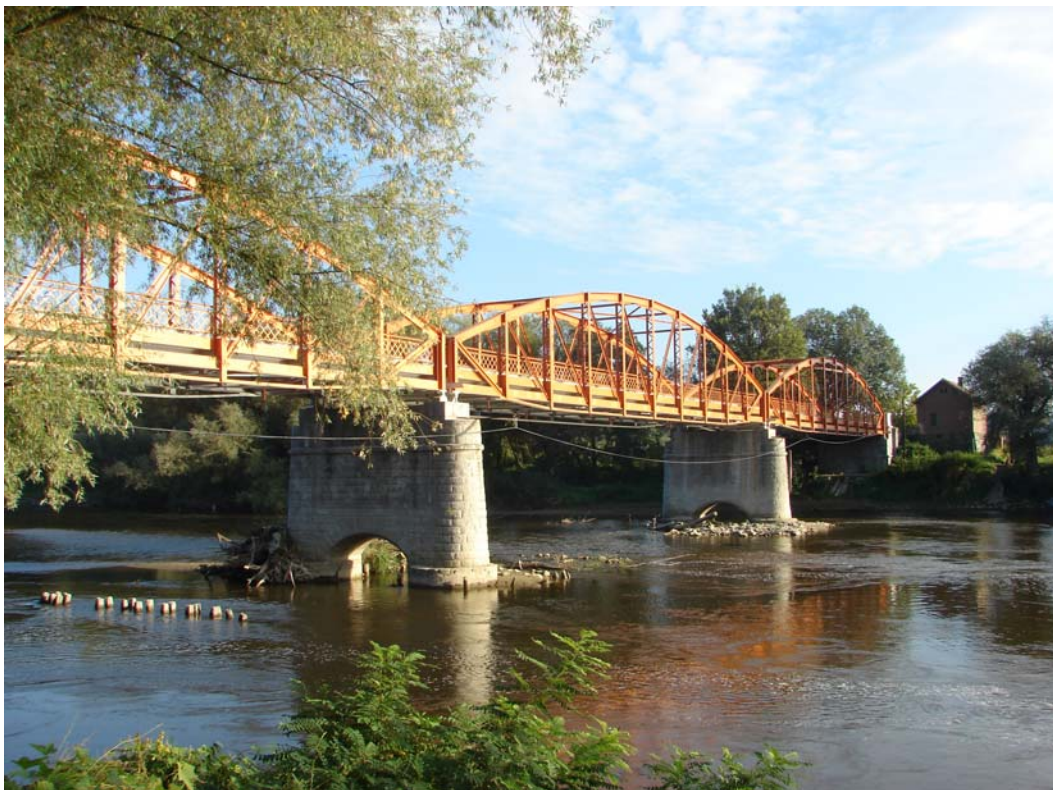
Fig.12 Savarsin Bridge after rehabilitation
