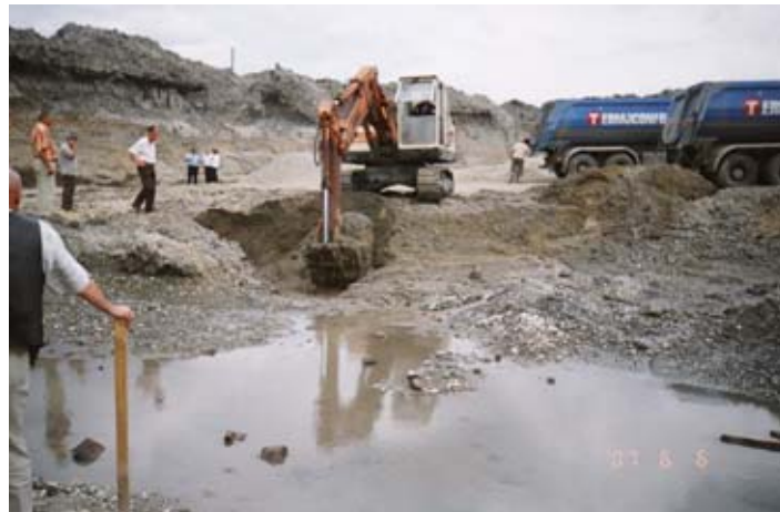
Fig. 2 The level of the groundwater at the beginning of the excavations
