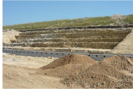
Fig.3 Slope excavation with joining steps
