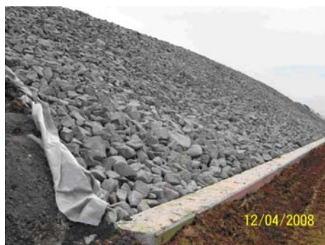
Fig.1 Slope stabilization with drainage mask km 35+160 – km 35+660
