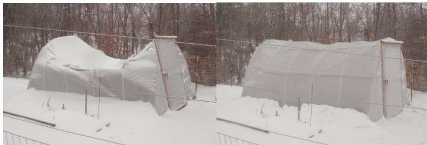
Figure 1: PVC tube greenhouse collapsed and after deformation[7]
