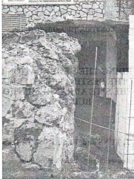
Fig. 1. – Appearance of earth filling behind the retaining wall.
