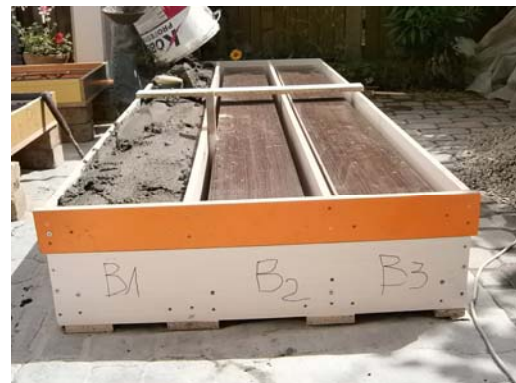
Fig. 1. Snapshots during execution of nonrecuperable shuttering for lintels
