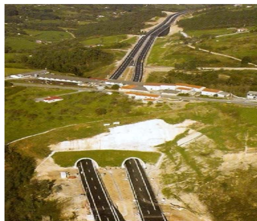
Fig. 6. Road tunnel spacing for each direction
