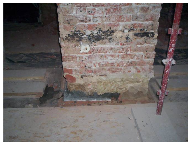
Fig. 10 Comer method applied at an interior column.
