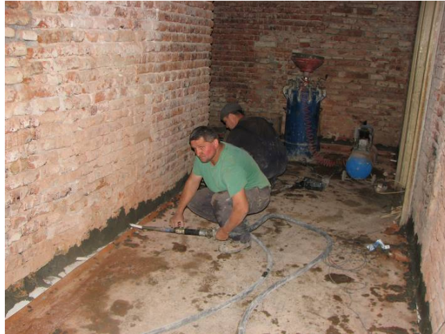
Fig. 11 Cement mortar injection into the cut.
