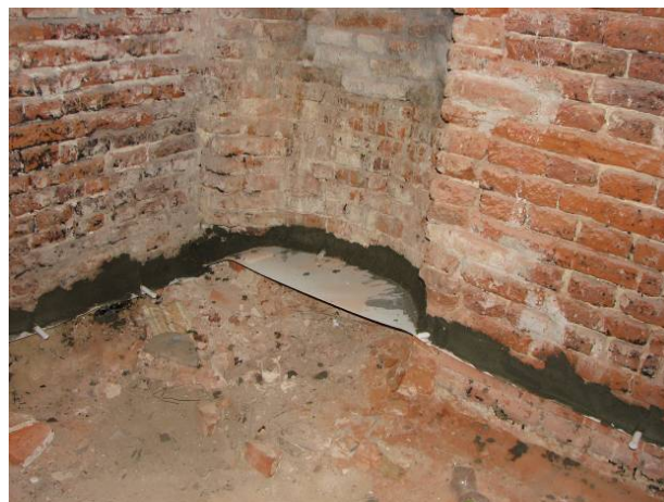
Fig. 9 Placing insulated sheet and wedges into an interior wall cut.
